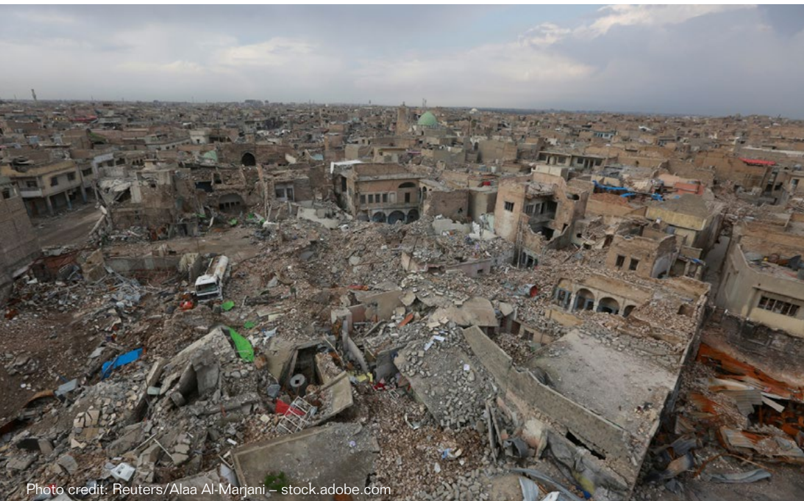
A general view of destroyed buildings in the old city of Mosul. Photo taken on 24 February 2018.
