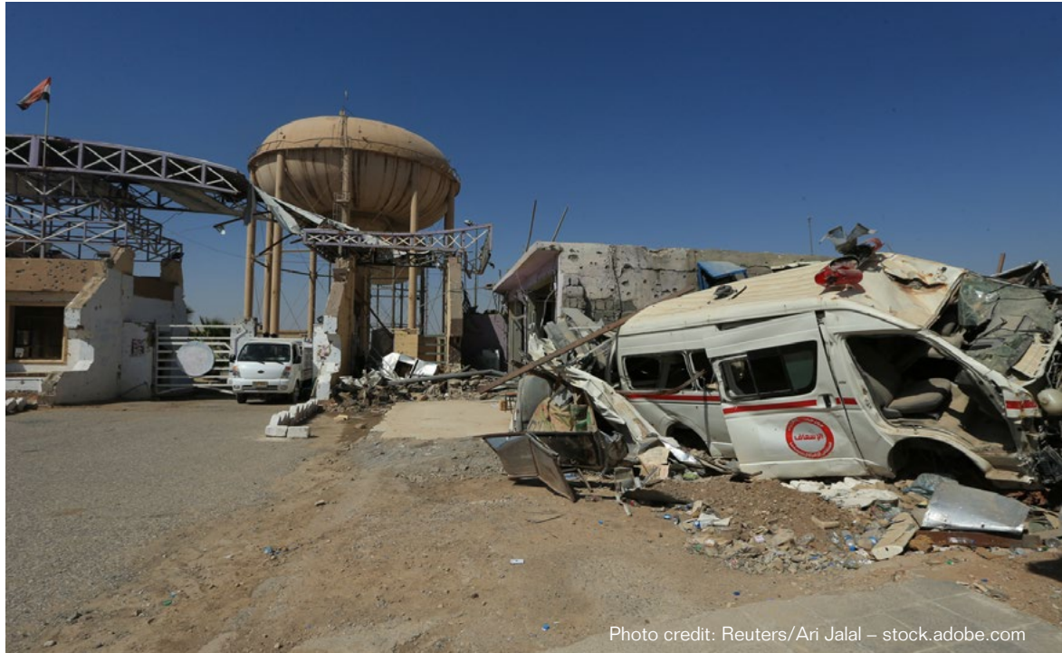
A view of the Republican hospital destroyed gate at the medical city in Mosul. Photo taken on 10 July 2018.
